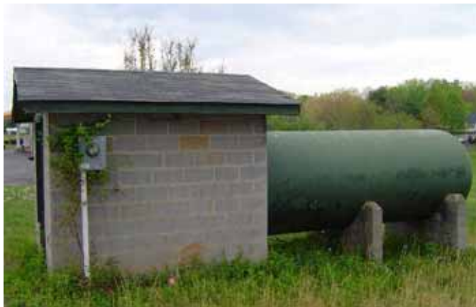
Figure 1: Typical Small Water System Well House, Storage Tank, and Disinfection System (Chlorination)
