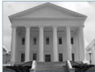
Renovation of the Virginia State Capitol was completed in 2007, the 400th anniversary of the founding of Jamestown
